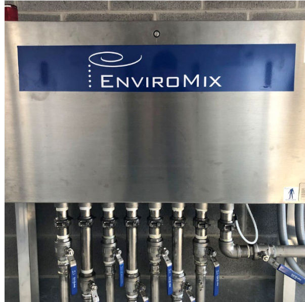
Zombie valve module (ZVM), with throttling valve and individual air control valve (ACV) isolation valves
