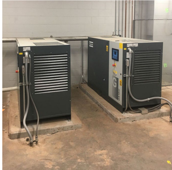
Compressors to be located indoors for weather protection and ease of maintenance
