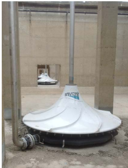
Figure 1: HYPERCLASSIC® -Mixing and Aeration System in Manchester, CT
