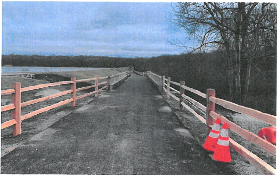
Path at entrance from North Main Road.
