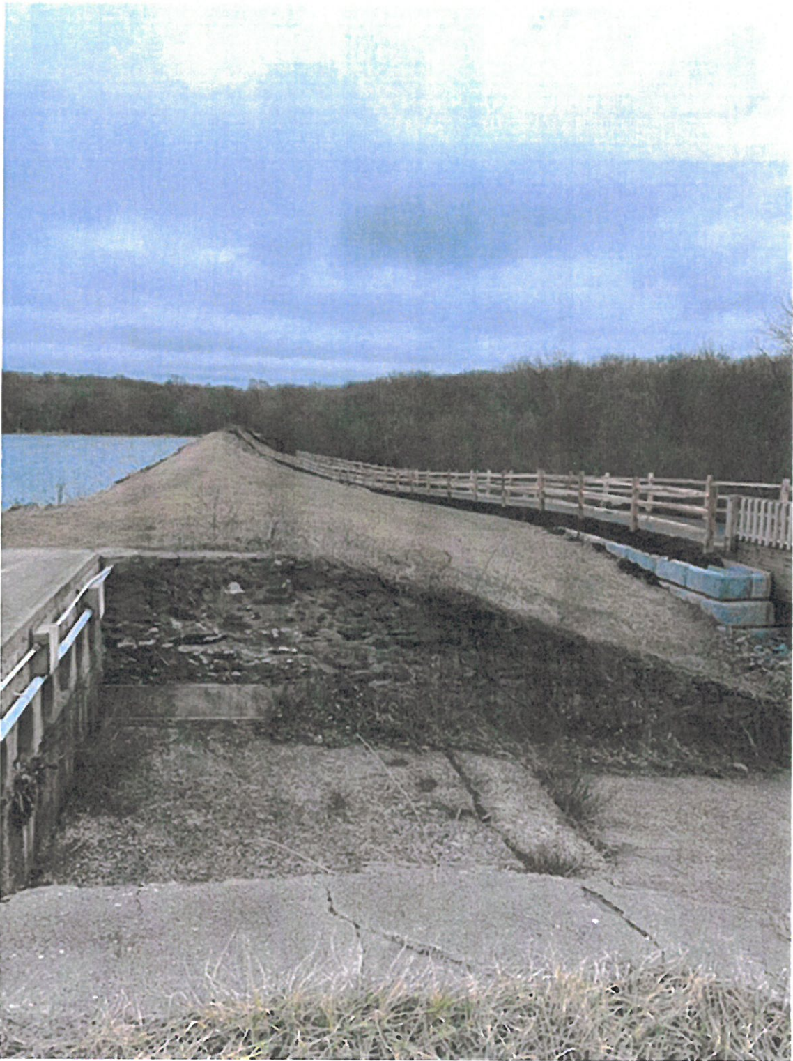
Path along the Reservoir and Dam
