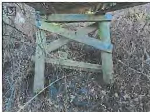
PILE BENT B2 TO BE SISTERED
